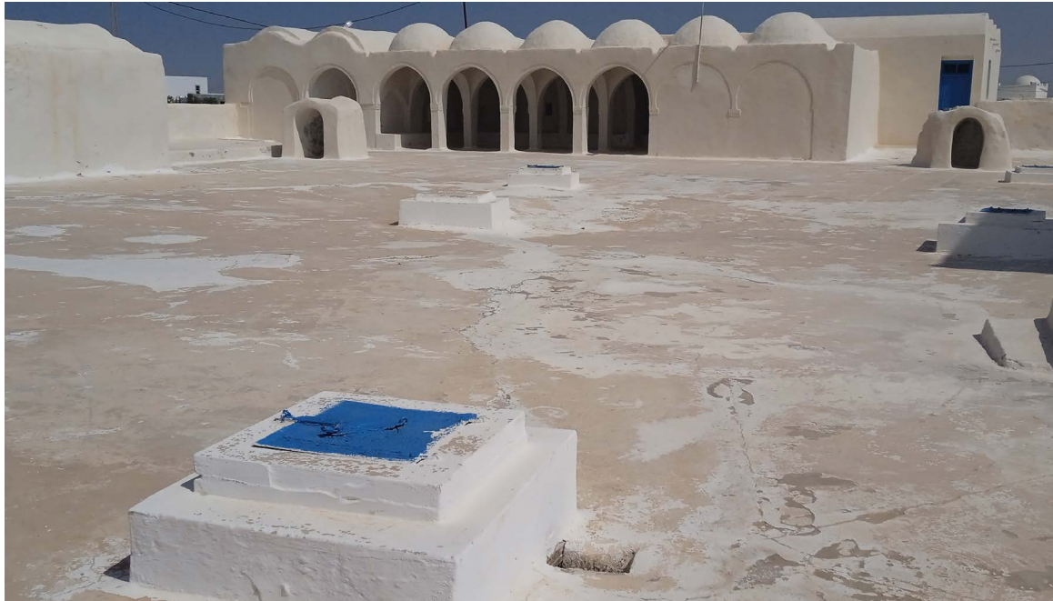
^ Fig. 2 Courtyard of a mosque, Djerba, where rainwater is collected and stored. This photograph depicts several underground cisterns employed for rainwater collection (Source: Sarra Ben Youssef, 2023).
