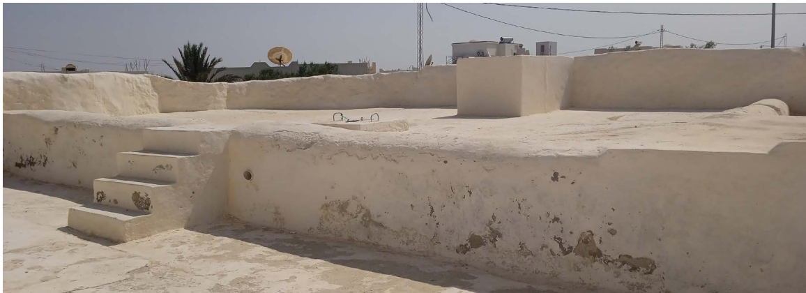
^ Fig. 4 A public rainwater cistern for charitable purposes, Feskia type (rectangular with impluvium) (Source: Sarra Ben Youssef, 2023).
