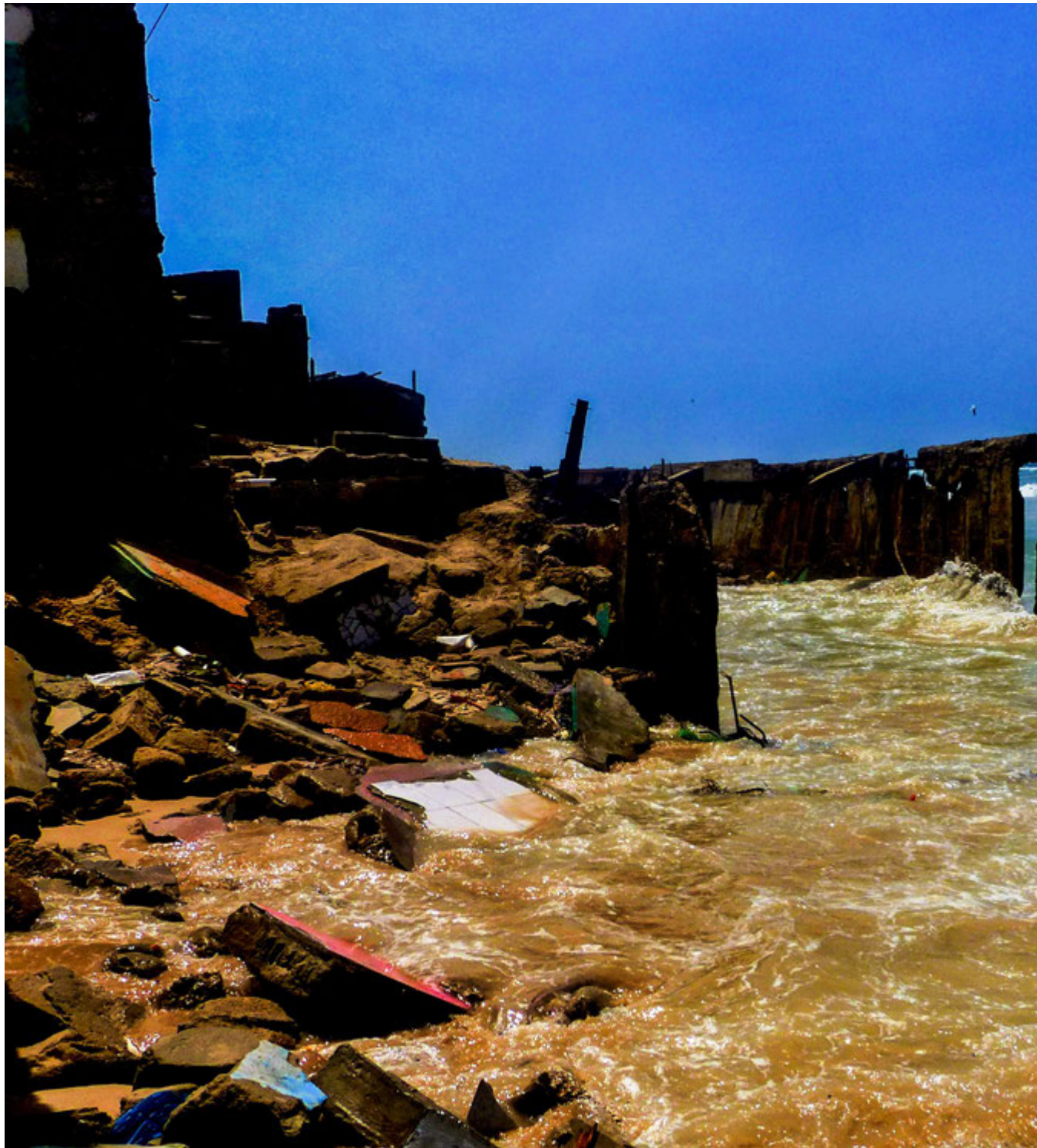
^ Fig. 3 Houses destroyed by erosion along the coast of the Island of Saint-Louis (Source: Abdoulaye Toure, 2021).
