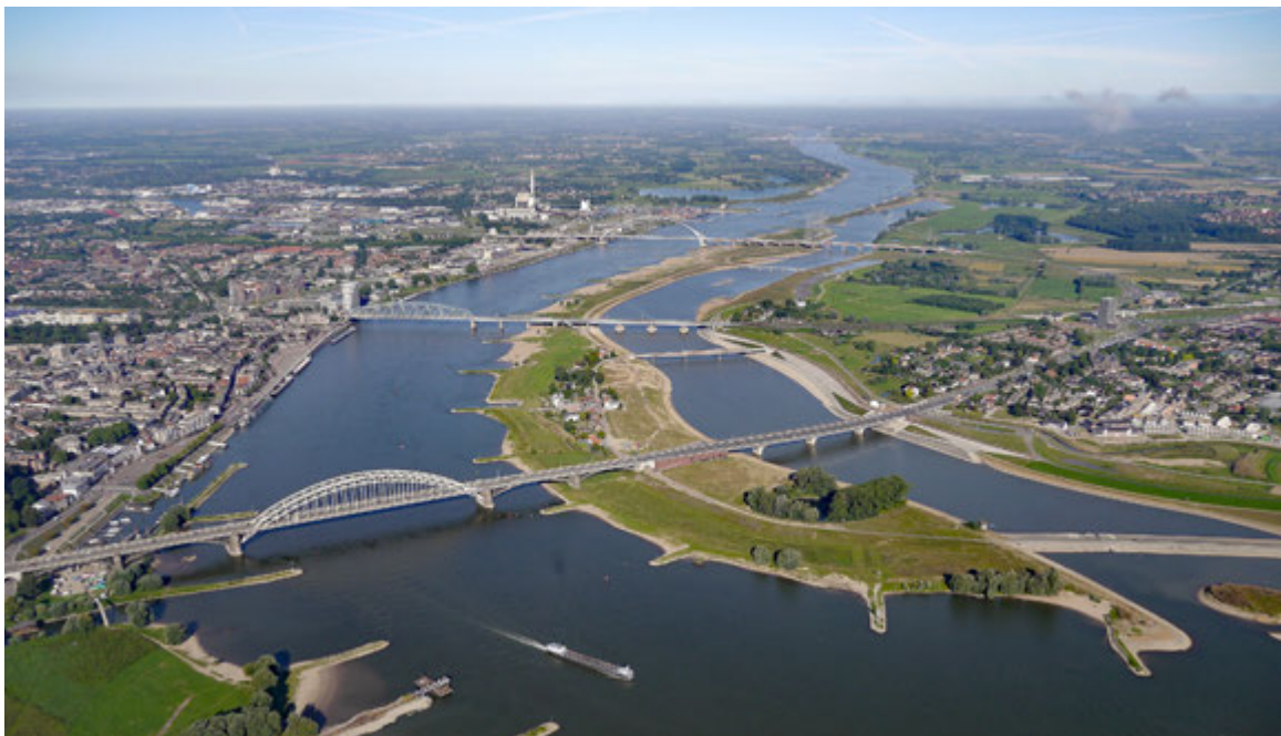
^ Fig. 6 Secondary canal in the Waal River at Nijmegen, constructed as part of the Room for the River program (Source: Johan Roerink, via Aeropicture.nl).
