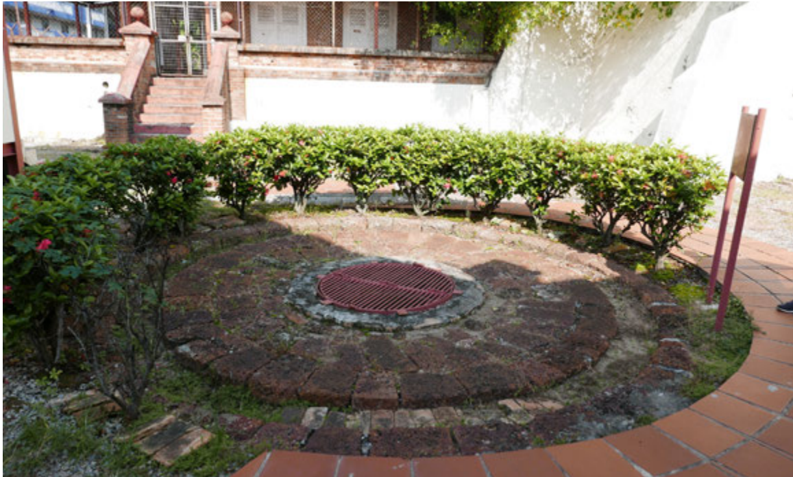
^ Fig. 2 One of the remaining well structures from the Dutch era in Malacca at the Stadthuys complex shows a mixed use of Portuguese laterite stone for drainage and the Dutch addition of brickworks for defense (Source: Queenie Lin, 2018).
