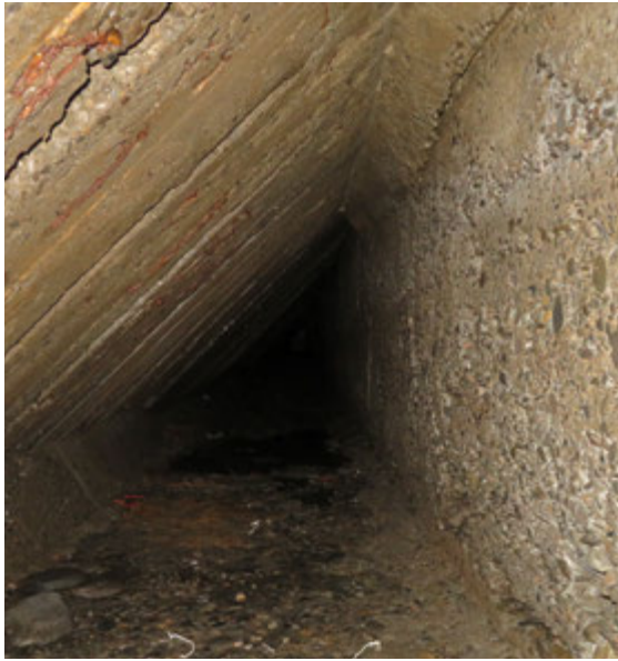
^ Fig. 3 The interior of the underground weir in the EICS (Source: Szu-Ling Lin and Cheh-Shyh Ting).
