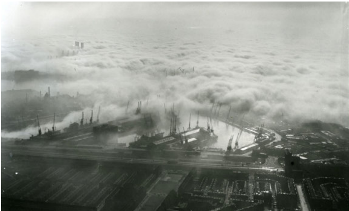
^ Fig. 3 Aerial photo of old Mathenesse and Merwehaven in 1971, with cranes and gasworks on theright (Source: Group A, 2020).
