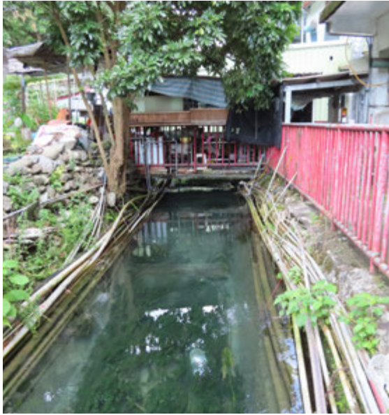
^ Fig. 6 The pipes covering the conveyance waterway of the EICS (Source: Szu-Ling Lin and Cheh-Shyh Ting).
