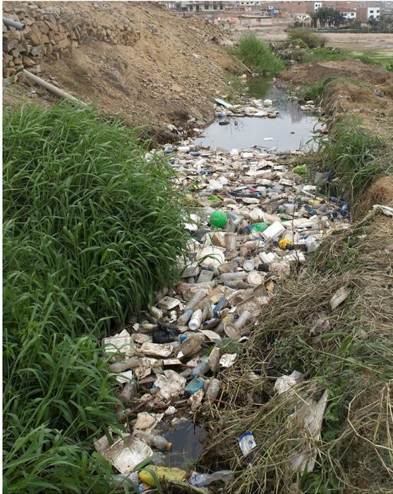
^ Fig. 5 Illegal dumping of waste is one of the major problems in functioning of the canals (Source: Javier Lizarzaburu).
