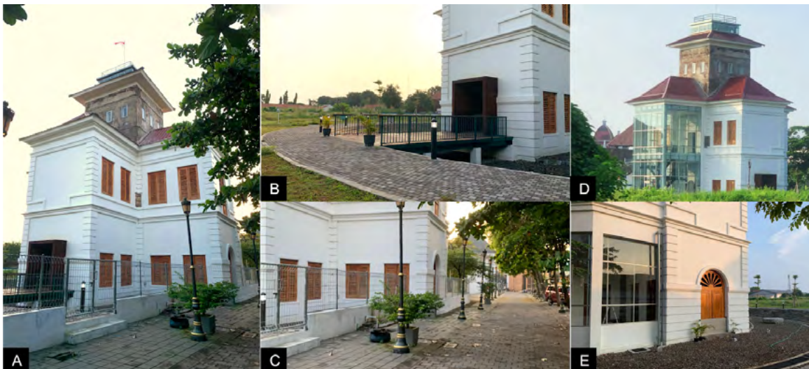
^ Fig. 4 Views of the harbormaster towers in Semarang after adaptive reuse: (A) overall view; (B) main entrance; (C) renovated pedestrian walkway; (D) curtain-wall intervention restoring the tower's original configuration; (E) glass addition distinguishing old structure from new (Source: Ricky Purbaya, 2024).
