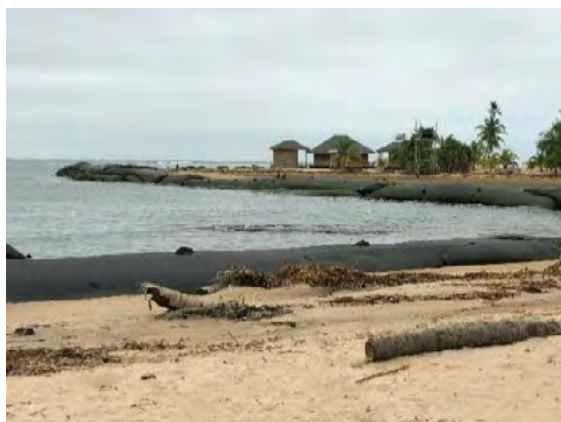
^ Fig. 6 Erosion control with sand tubes (Source: Rhoda Osei-Nkwantabisa, 2022).
