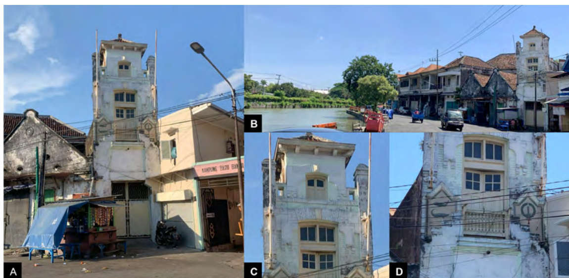
^ Fig. 6 Views of the harbormaster tower in Surabaya: (A) façade; (B) view toward the Kalimas River; (C) masonry detail; (D) emblems of Surabaya (left) and Batavia (right) (Source: Ricky Purbaya, 2024).
