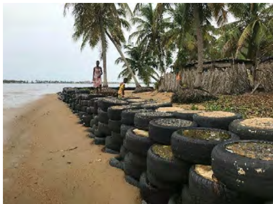
^ Fig. 5 Erosion control with car tires (Source: Rhoda Osei-Nkwantabisa, 2022).
