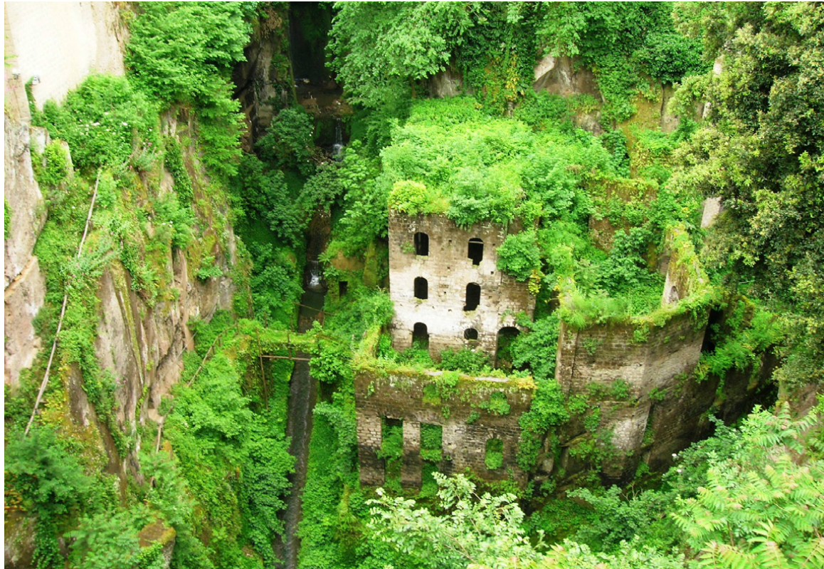
^ Fig. 4 Vallone dei Mulini, Sorrento – Costiera Amalfitana, UNESCO Cultural Landscape, Italy. A natural canyon where watermills began operating in the thirteenth century, showing the interaction between geomorphology, vegetation and historic hydraulic systems for paper production; the site vividly illustrates the sophisticated pre-industrial water network that sustained Amalfi's paper industry within a dramatically sculpted landscape (Source: Mentnafunangann. CC BY-SA 3.0, via Wikimedia Commons).
