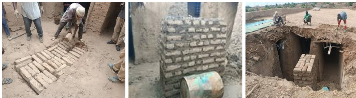
^ Fig. 3 Repair work on the roof of the men's mosque after the 2024 collapse (Source: Mamadou Samaké, 2024).
