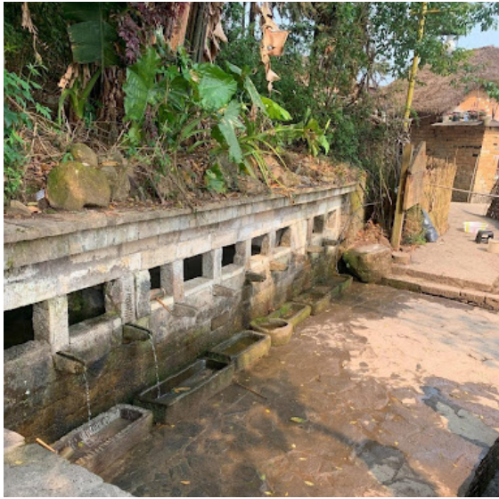
^ Fig. 3 A water diverting and management structure in a village in the Honghe Hani Rice Terraces (Source: Tianchen Dai, 2024).
