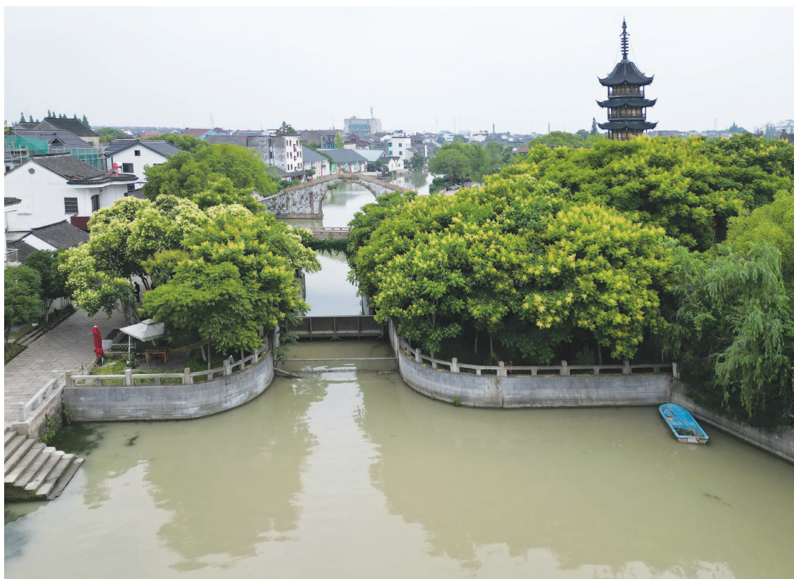
^ Fig. 6 The addition of modern sluices between the polders forms weiqu . The entrance of Zhenze is now demarcated by a sluice (added in 1997) near the ancient Yuji Bridge (Source: Wei Lei, 2023).
