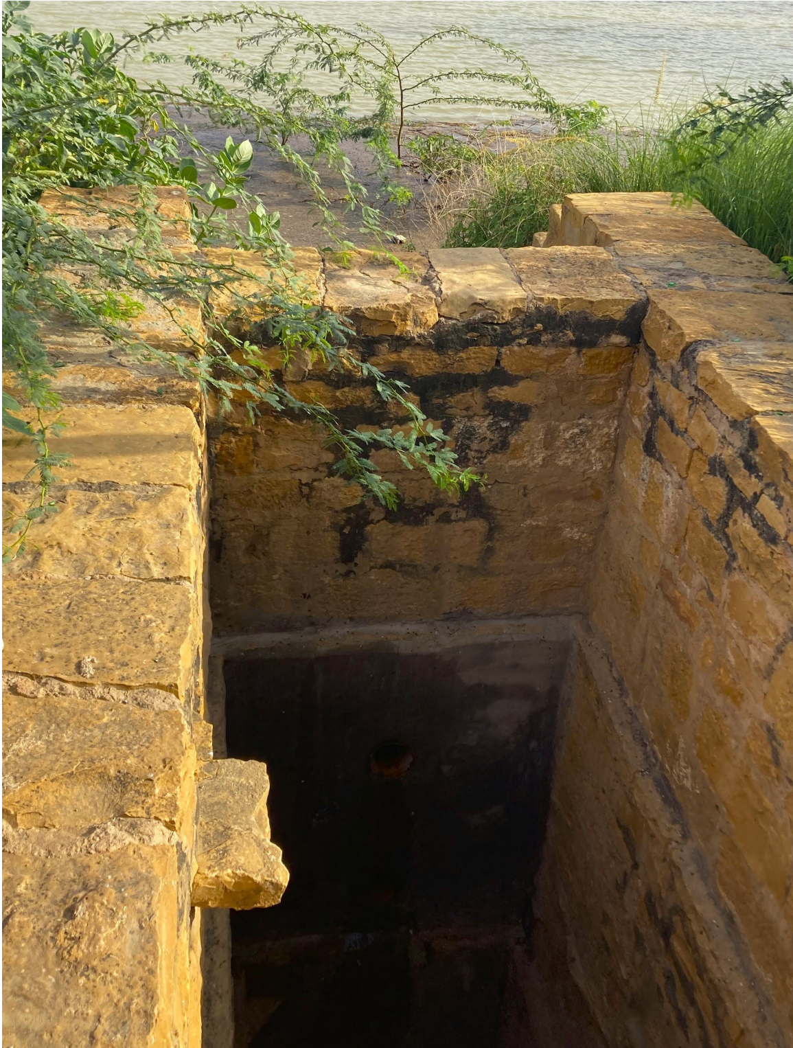
^ Fig. 6 Outlet shaft at the Bada Bagh Khadeen (Source: Pierantonio La Vena, 2023).
