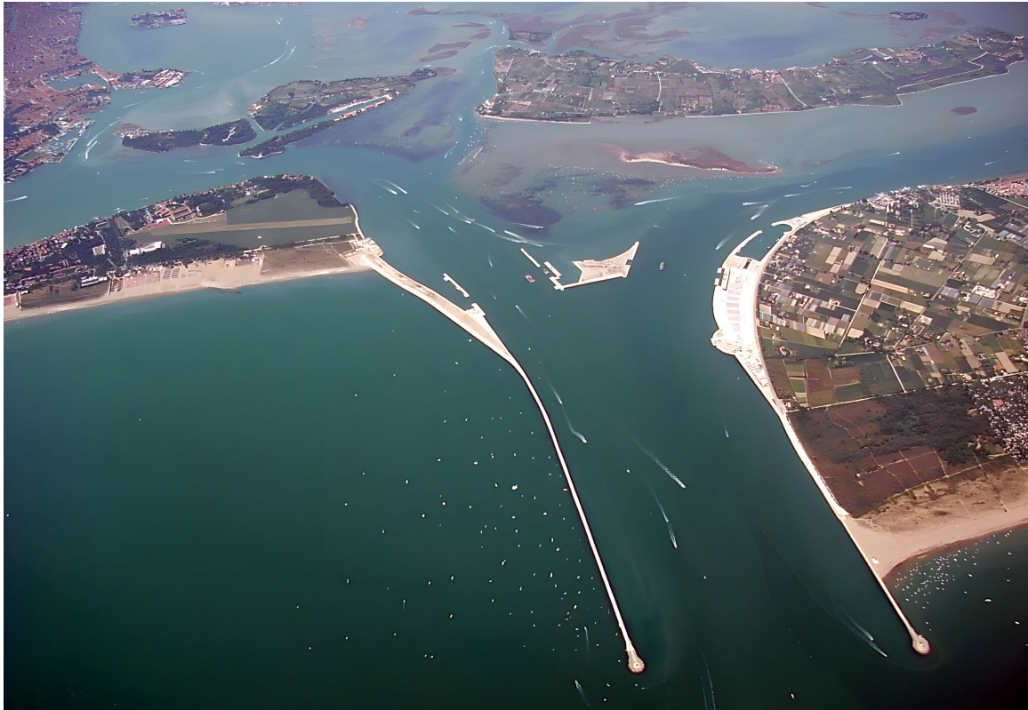
^ Fig. 10 Aerial view of the MoSE project in Venice, Porto di Lido (channel north of Lido) in mid-2009 (Source: Chris 73, 2009. Wikimedia Commons, CC BY 3.0).
