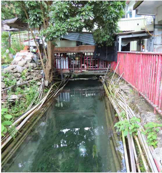
^ Fig. 6 The pipes covering the conveyance waterway of the EICS (Source: Szu-Ling Lin and Cheh-Shyh Ting).
