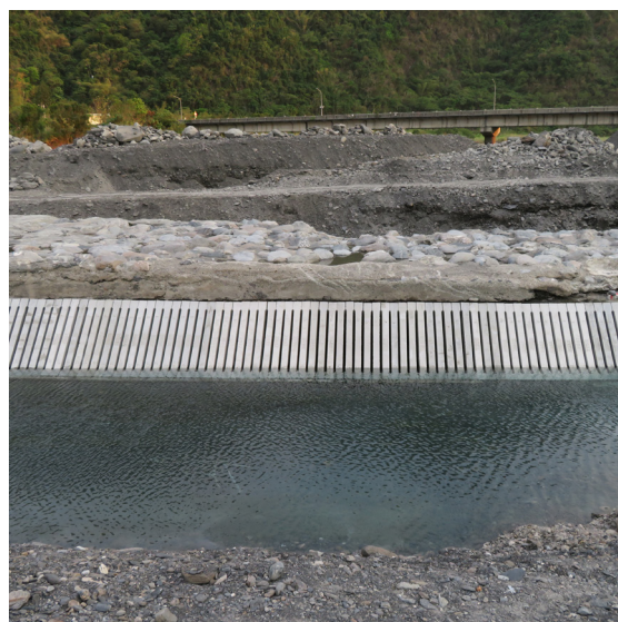
^ Fig. 5 The construction of the underground weir in EICS (Source: Szu-Ling Lin and Cheh-Shyh Ting).
