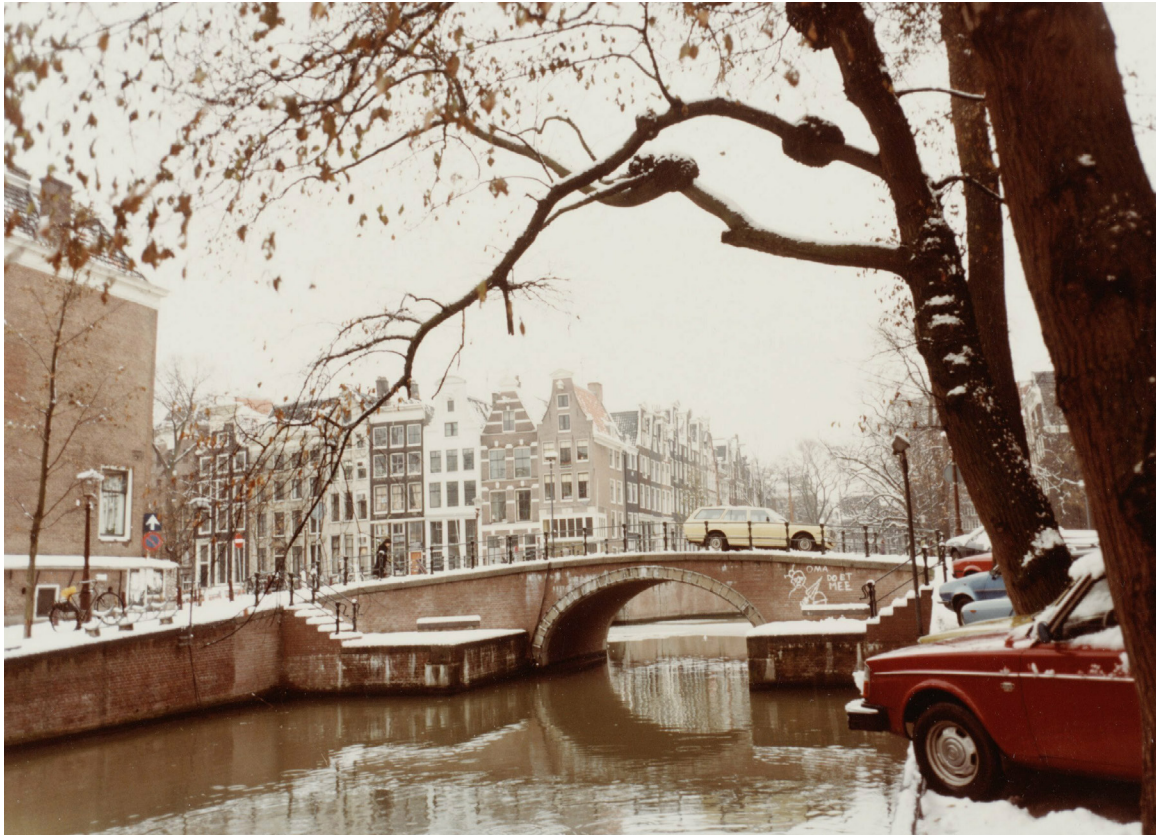
^ Fig. 5 Bridge 44, Leidsegracht, where the platforms show traces of a lost function: closing doors were operated to force flow in the flushing scheme between 1663 and 1872 (Source: Stadsarchief Amsterdam, B00000024728).
