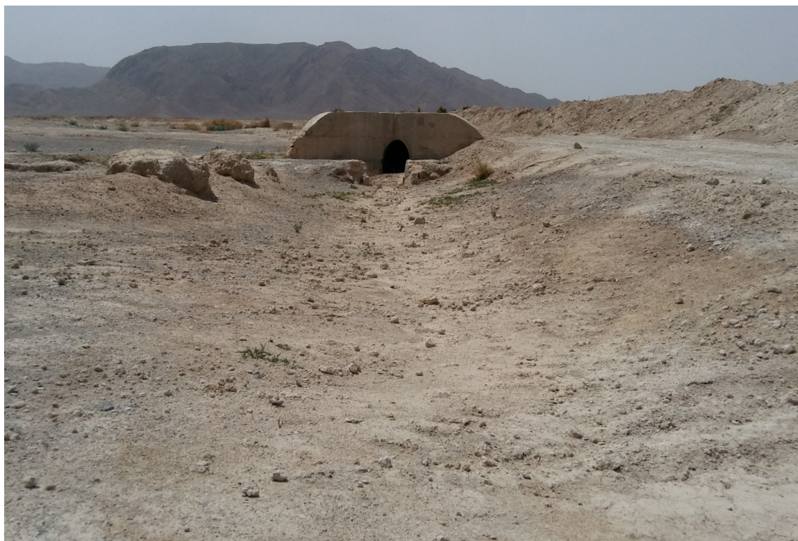
^ Fig. 4 The qanat of Cheshme Chāhak in the basin downstream, which dried up after groundwater overexploitation in the basin upstream (Source: Majid Labbaf Khaneiki and Abdullah Saif Al-Ghafri 2018).
