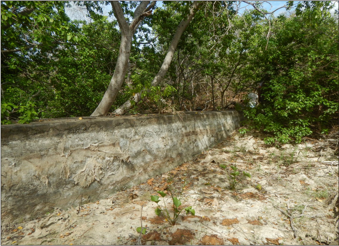
^ Fig. 2 Stone and earthen dams were built in the rooi-streambeds for water retention and to prevent water from running off to sea. (Source: John Dohmen, 2017. CC BY-NC).
