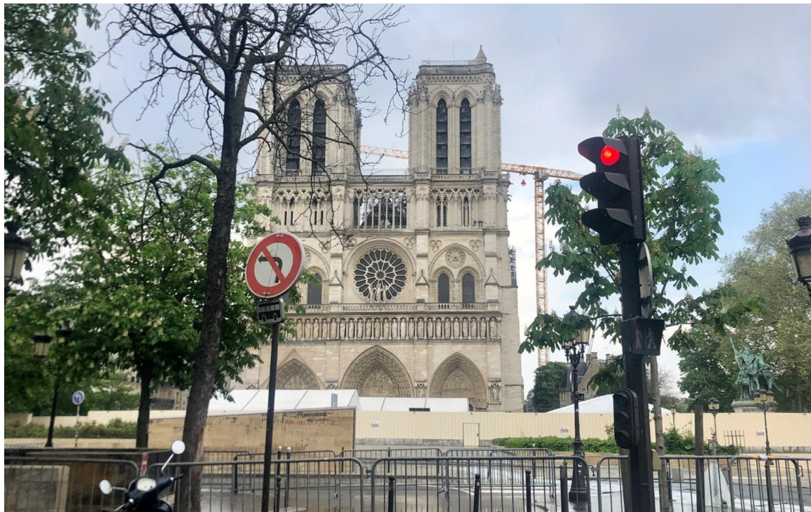
^ Fig. 5 The cathedral forcourt in construction, Notre Dame de Paris (Source: Emmanuelle Lallement, 2022).
