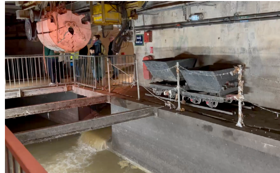
^ Fig. 12 Some underground galleries of different sizes that are part of the sewage system of Paris are accessible as part of the Paris Sewer Museum (Source: Carola Hein, 2025).
