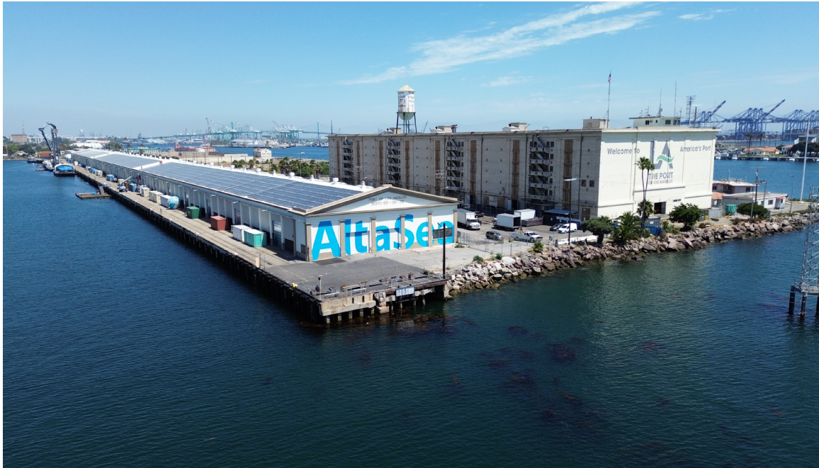
^ Fig. 3 AltaSea West Campus with 180,000 sq ft (16,723 m 2 ) of renovated warehousing equipped with solar panels (Source: AltaSea, 2024).
