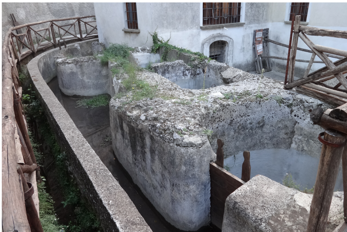
^ Fig. 7 Amalfi Paper Museum – Costiera Amalfitana, UNESCO Cultural Landscape, Italy. Wooden sluice gates regulating the water-powered papermaking process, exemplifying the artisanal hydraulic ingenuity that defined the Amalfi Coast’s long-standing role in European paper production (Source: Derbrauni, 2014. CC BY-SA 4.0, via Wikimedia Commons).
