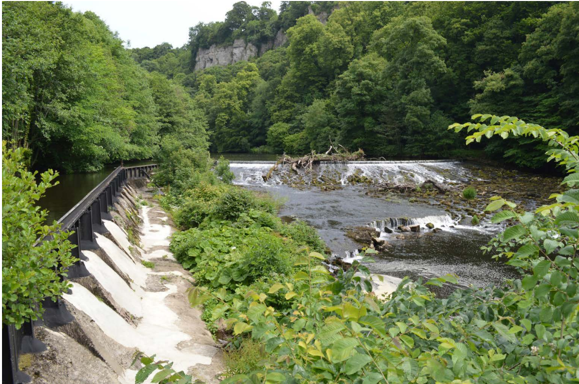
^ Fig. 2 Derwent Valley Mills – UNESCO Industrial Heritage (United Kingdom). View of the River Derwent weir at Masson Mills, part of the hydraulic system that powered textile factories shaping the factory model of the Industrial Revolution. Current studies explore its reuse for micro-hydropower within heritage frameworks (Jackson 2024) (Source: John M, 2013. CC BY-SA 2.0, via Wikimedia Commons).
