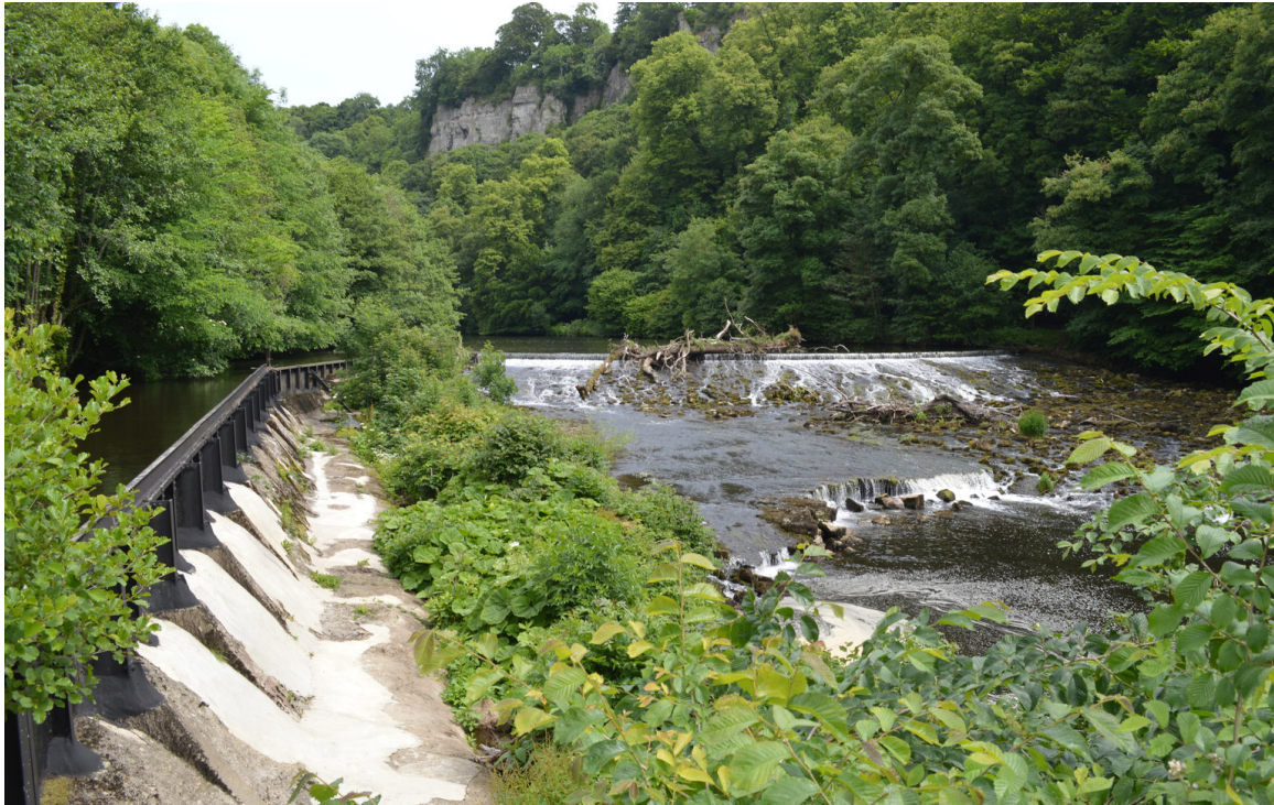
^ Fig. 2 Derwent Valley Mills – UNESCO Industrial Heritage (United Kingdom). View of the River Derwent weir at Masson Mills, part of the hydraulic system that powered textile factories shaping the factory model of the Industrial Revolution. Current studies explore its reuse for micro-hydropower within heritage frameworks (Source: John M, 2013. CC BY-SA 2.0, via Wikimedia Commons).
