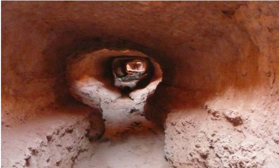
^ Fig. 5 Inside an underground desiccated gallery of a khattara light shines from above through the maintenance shafts. The gallery is tall enough for an average-sized person to stand up straight and wide enough to comfortably walk through. (Source: Cristiana Strava, 2010).
