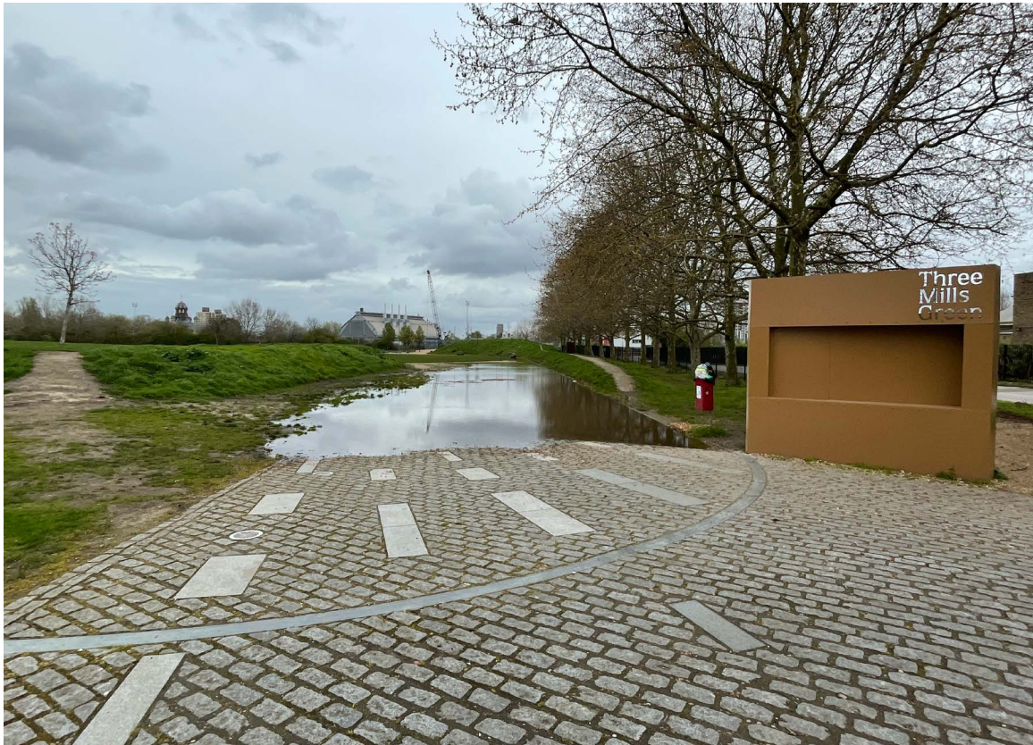
^ Fig. 3 Flooded footpath between Abbey Mill Pumping Station and the Lea (Source: Maia Brons, 2023).
