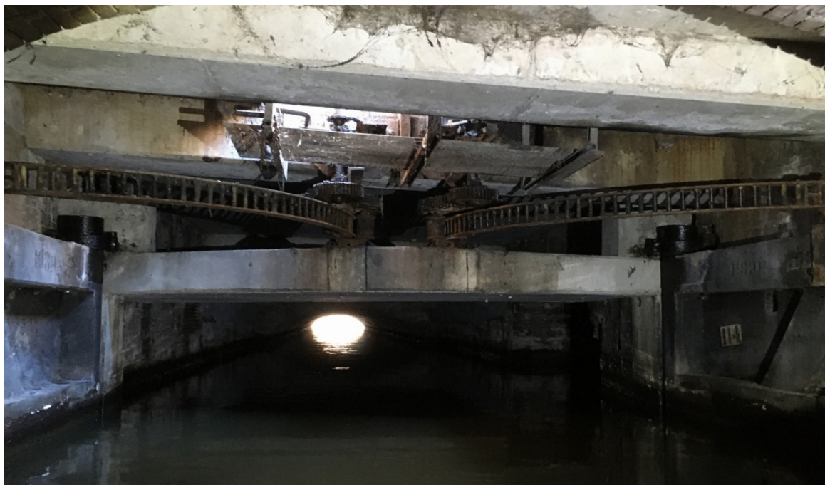
^ Fig. 5 1980 reconstruction of the closing doors in the underground canal under Nieuwmarkt, Amsterdam. The canal functions as a connection, eventually transporting water discharge from the Amstelland catchment in the direction of the North Sea. The closing doors protect the city from flooding when outside water levels are high (Source: Maarten Ouboter).
