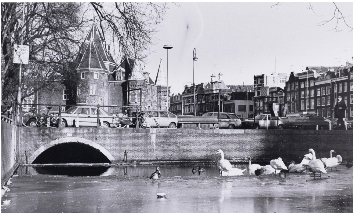
^ Fig. 3 Waag, seen from the Kloveniersburgwal in 1982. Development of the Nieuwmarkt square began in the early seventeenth century, extending the underground canal entrance (Source: B.P. Opschoor, Stadsarchief Amsterdam, OSIM00008002319).
