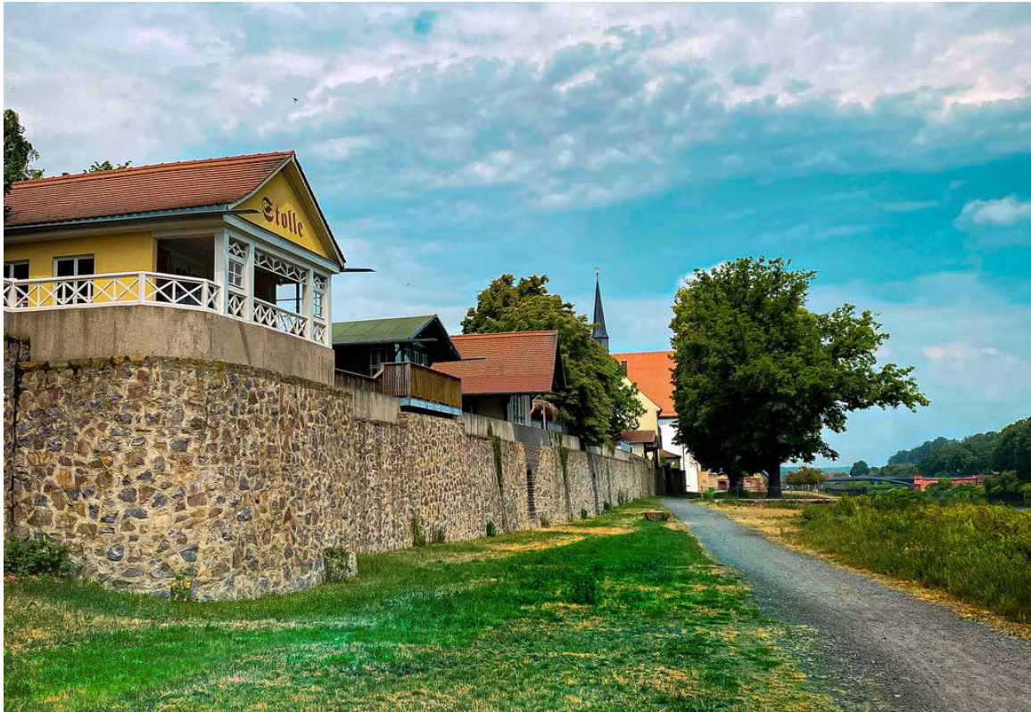
^ Fig. 5 Flood defense system in Grimma, Germany (Source: Sebastian Bachran, 2022).
